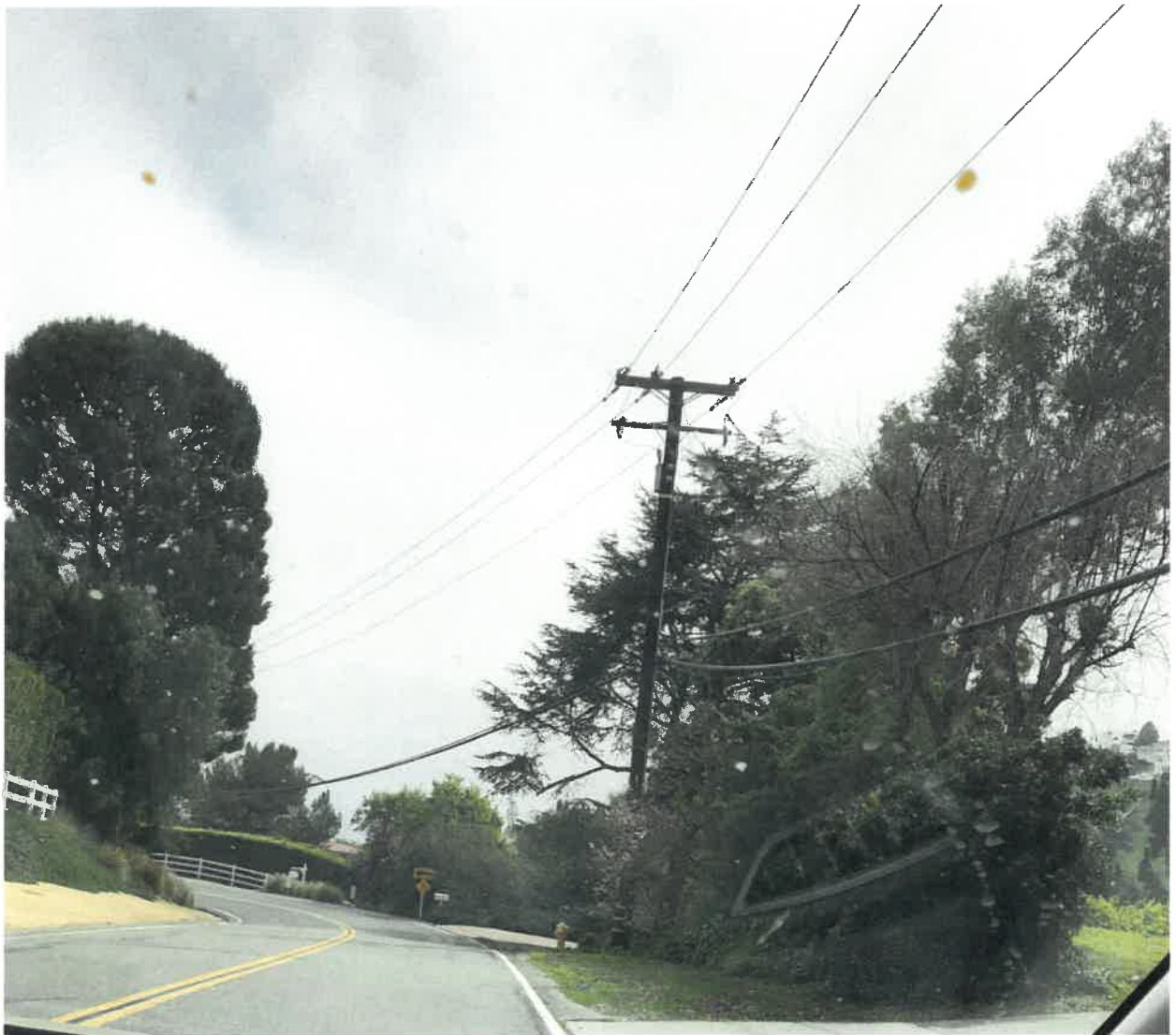
Existing Utility Lines Over Eastfield Drive (2019)
