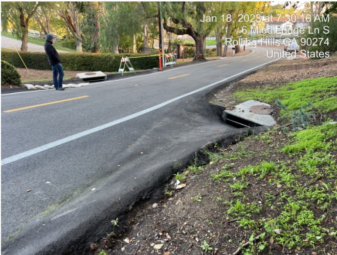
Photo 1 - Upstream 18" CMP at STA 8+17 (right side of photo) upstream 24" CMP at STA 7+84 (left side of photo).
