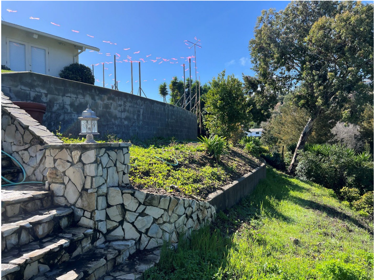
This photo was taken on the lower level of the building pad looking south
