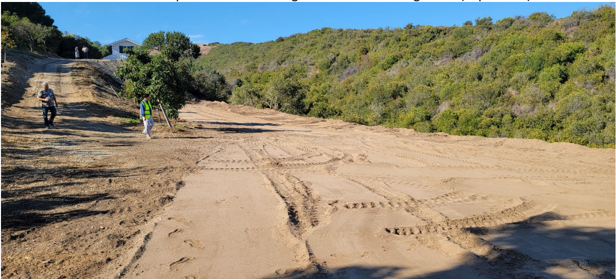
Bottom: Lower pad of 29 Middleridge Lane South looking south (Sept. 2022)
