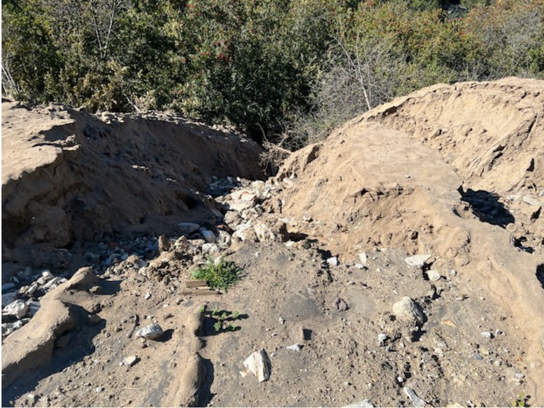
Top and bottom: Photos of erosion on lower pad of 29 Middleridge Lane South caused by rain (2/7/23)
