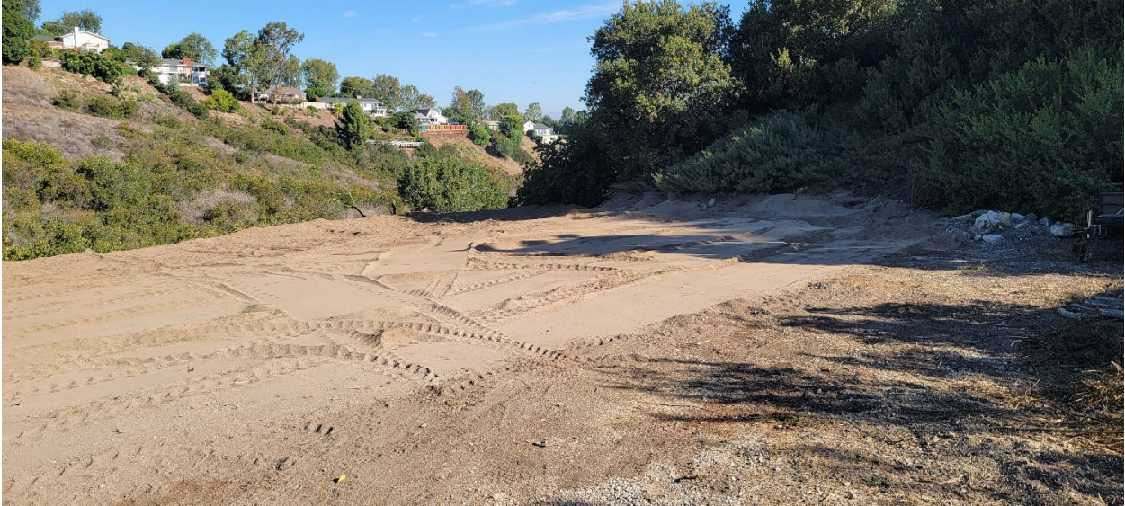
Top: Lower pad of 29 Middleridge Lane South looking north (Sept. 2022)
