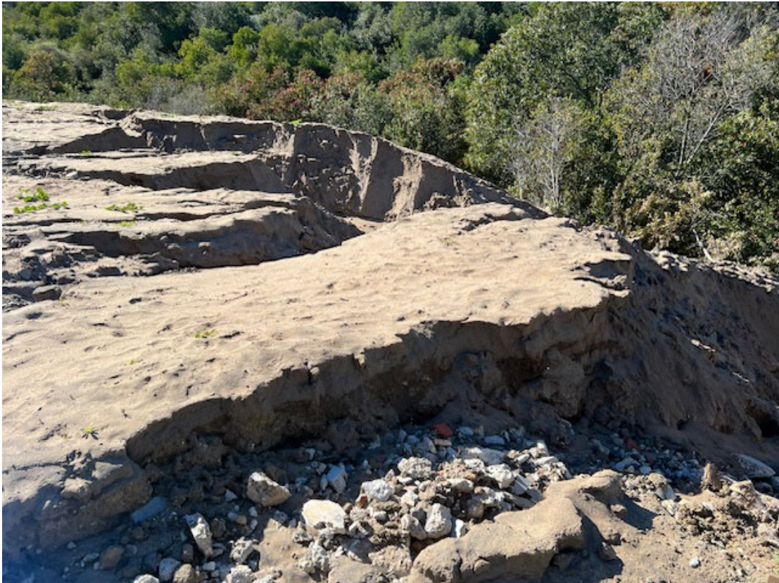
Top and bottom: Photos of erosion on lower pad of 29 Middleridge Lane South caused by rain (2/7/23)
