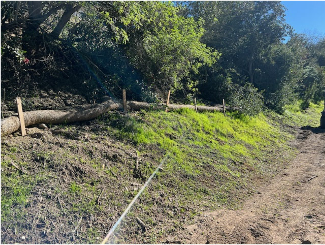
Top and bottom: Wattles to prevent further erosion onto Johns Canyon Trail (2/7/23)
