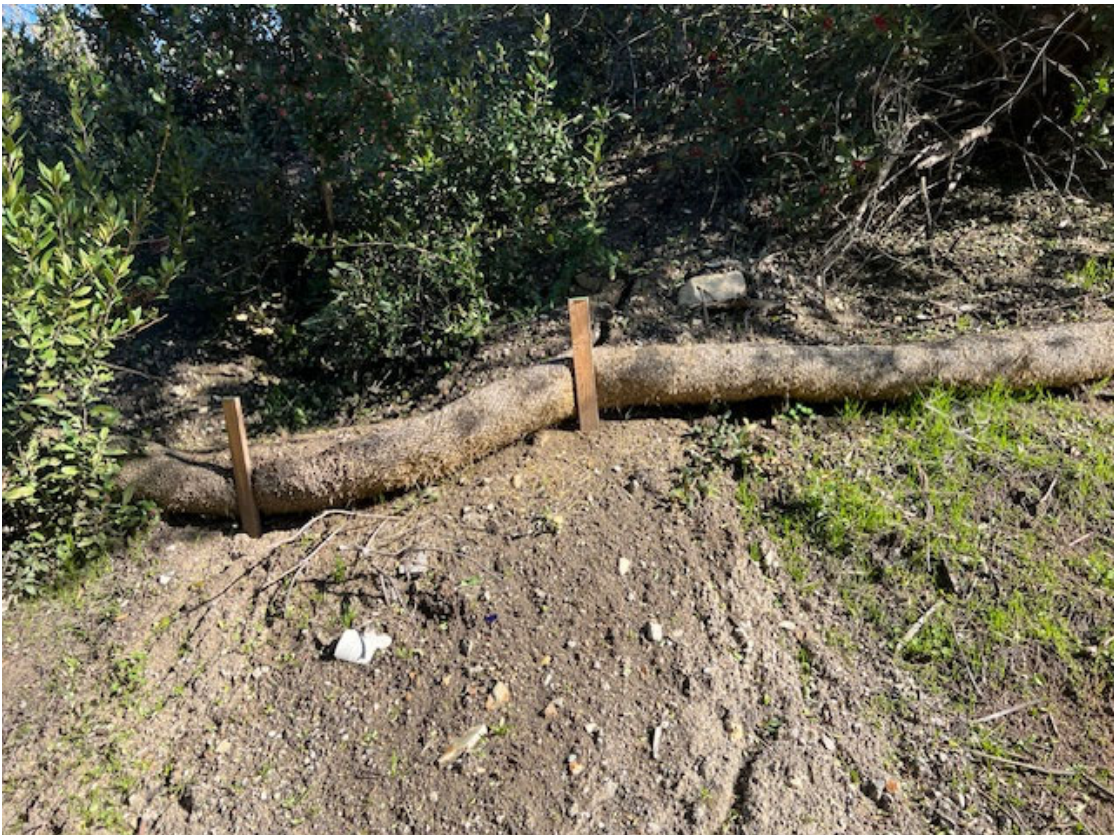
Top and bottom: Wattles to prevent further erosion onto Johns Canyon Trail (2/7/23)
