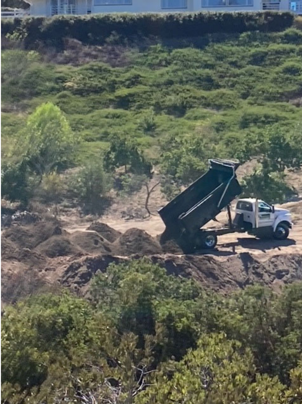
Close up of dump truck on lower pad of 29 Middleridge Lane South (Taken by resident, circa Sept. 2022)
