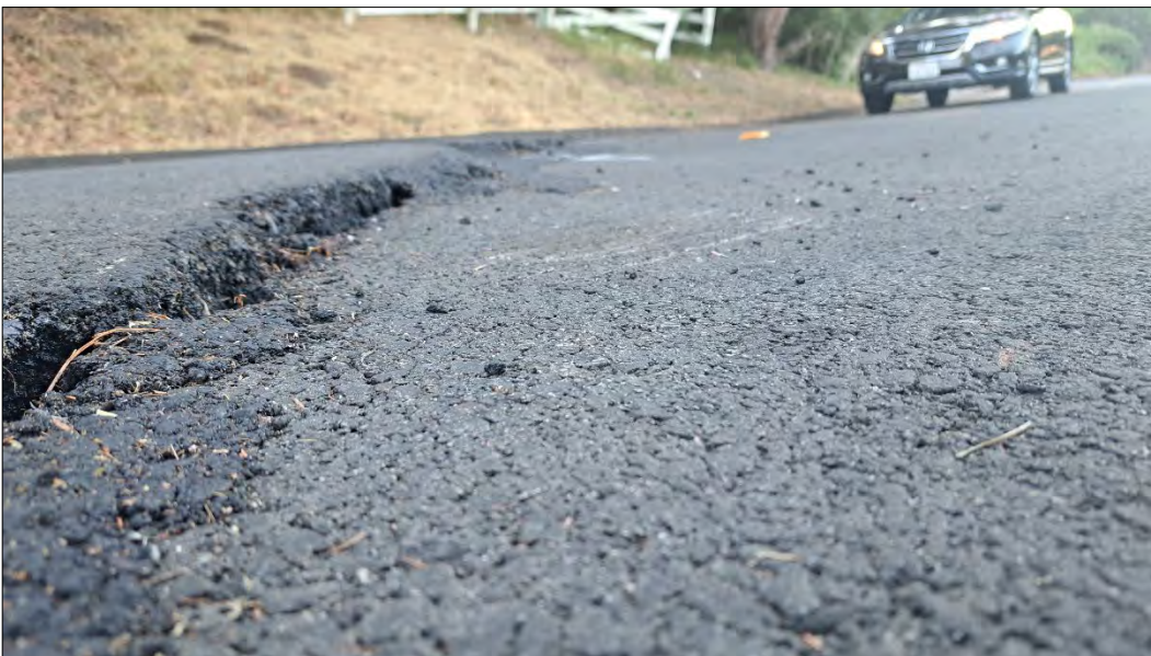
Figure 2: Crack and movement on Quail Ridge Rd. S.
