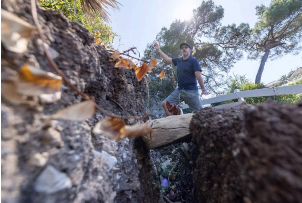
Figure 4: September 29, 2024 showing crack widening and vertical movement
