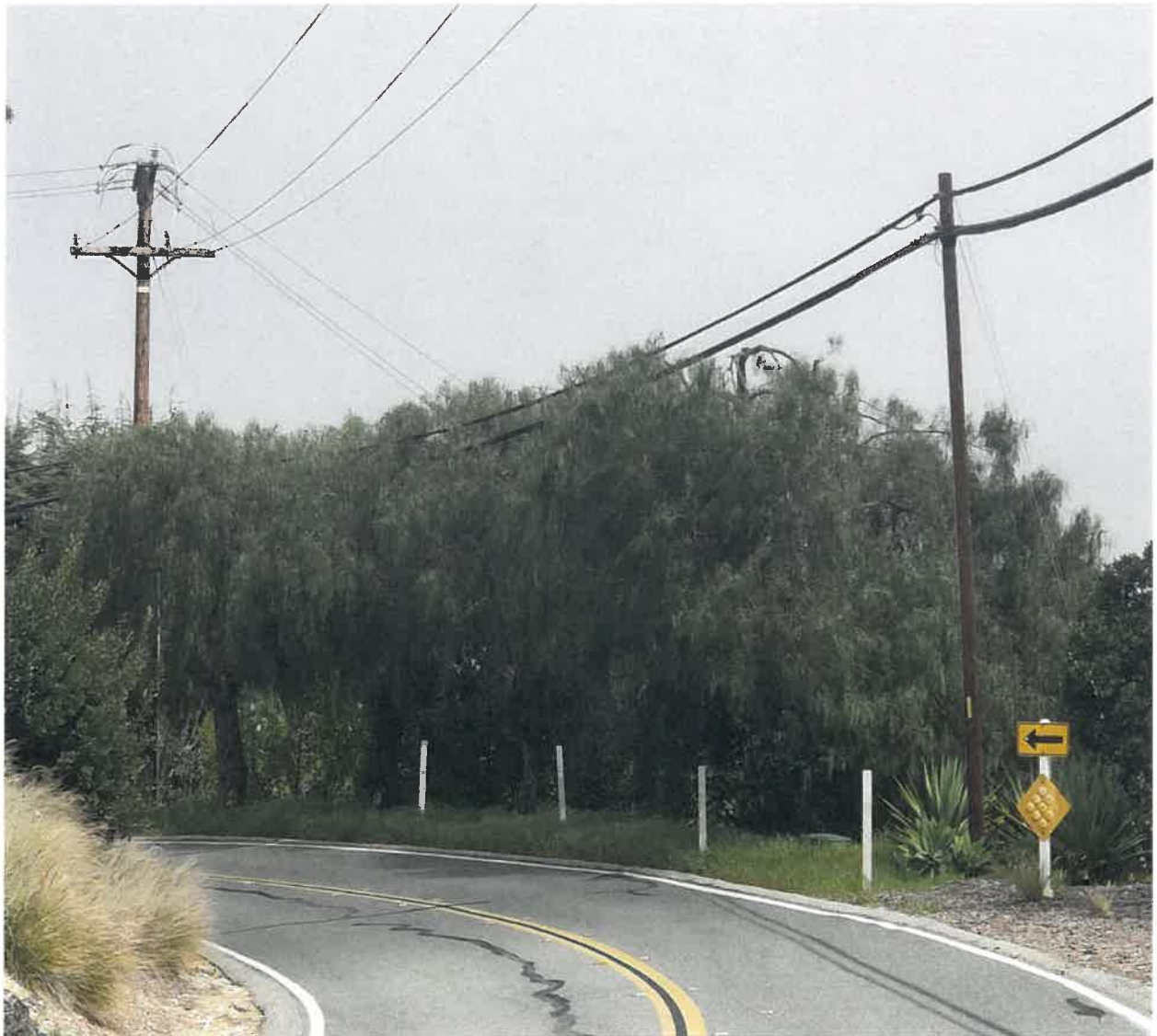
Existing Eastfield Drive Utility Lines Over Trees (2019)
