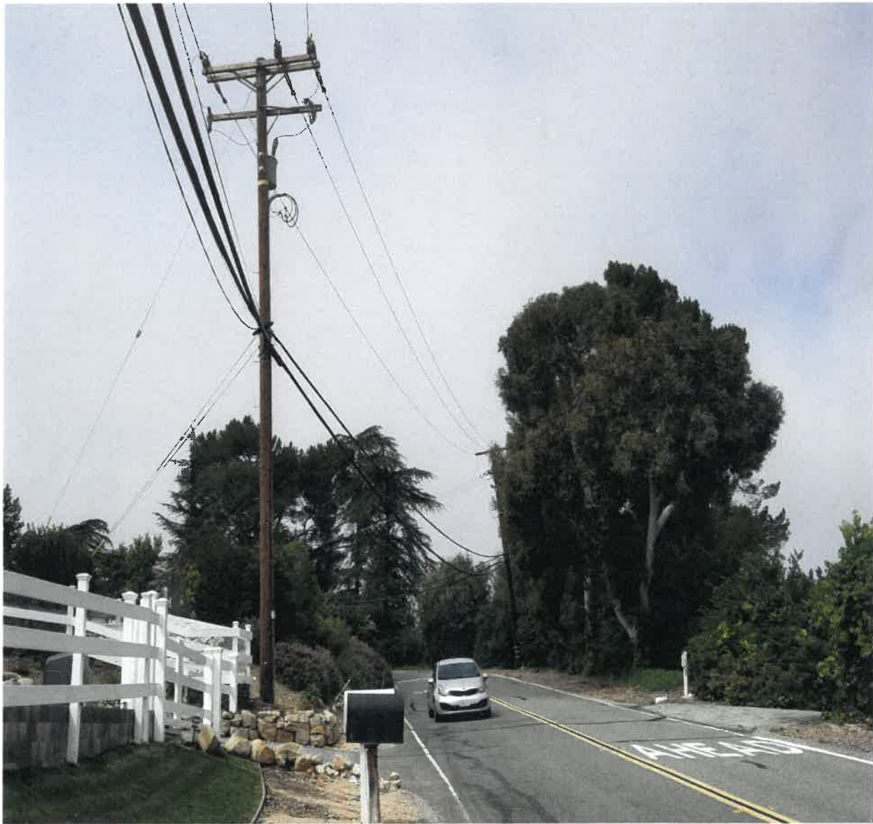
Existing Utility Lines on Eastfield Drive (2019)
