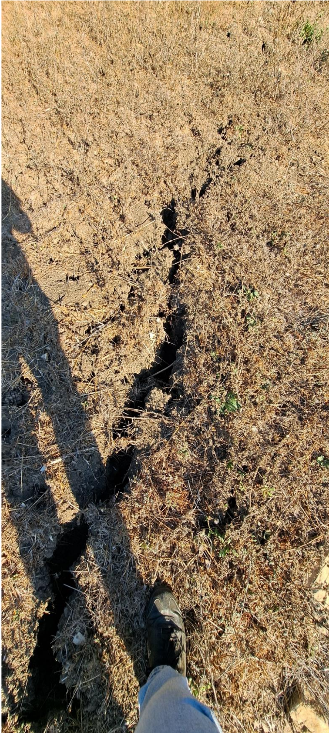
Figure 5: November 11, 2024 - Crack in Canyon Below 3 Quail Ridge S
