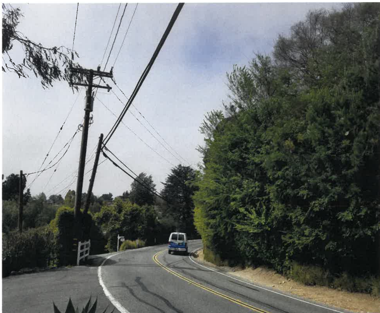
Existing Utility Lines on Eastfield Drive (2019)
