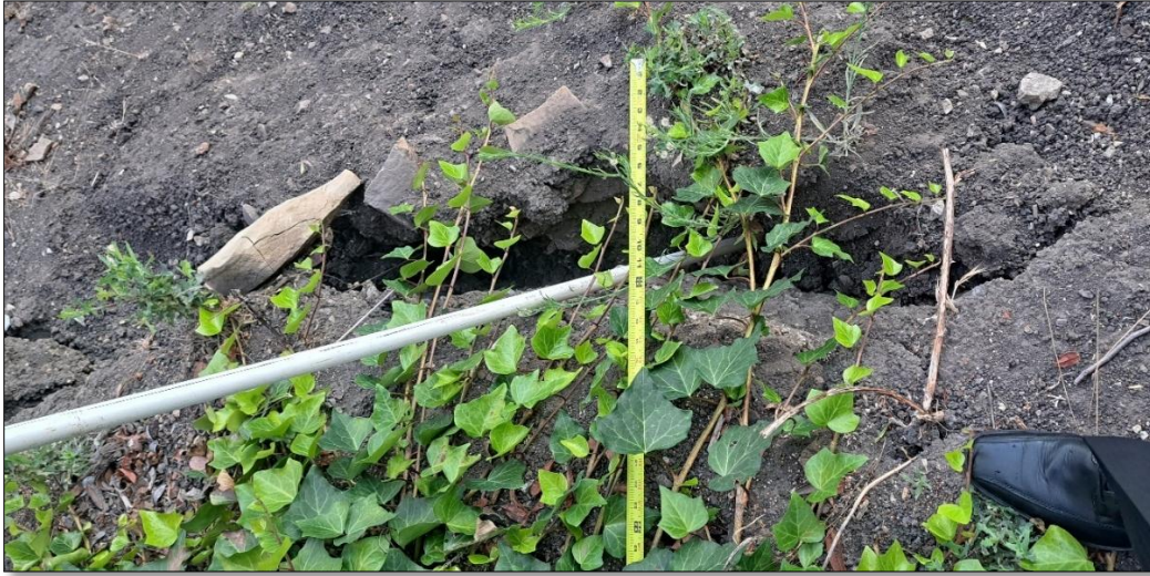
Figure 7: September 9, 2024 Crack between 3 and 5 Quail Ridge Rd. S.
