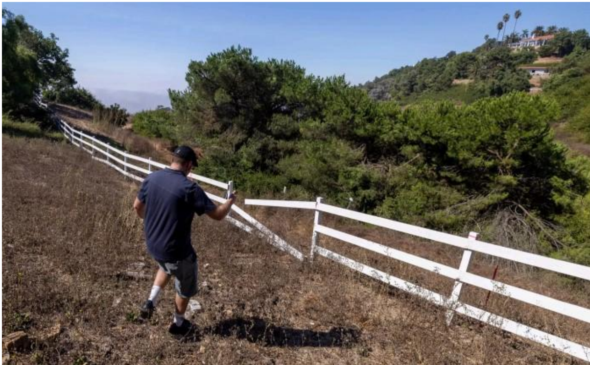
Figure 11: September 29, 2024 showing crack all the way through property and damaging fence
