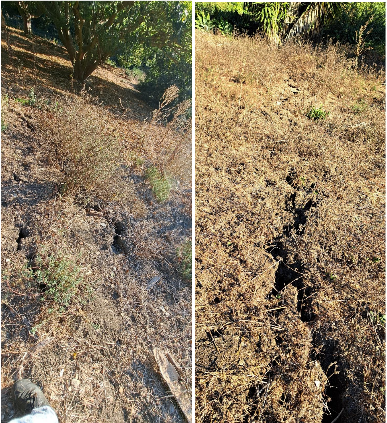
Figure 6: November 11, 2024 Crack and fracturing in canyon below 3 Quail Ridge Rd S
