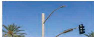
Small cells are low-powered, fiber-connected nodes that are usually located on existing structures like streetlights and utility poles.
