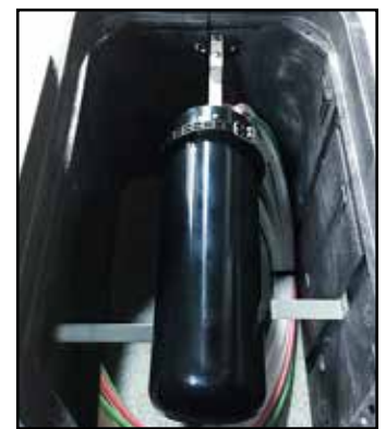
90° Splice closure mounting
